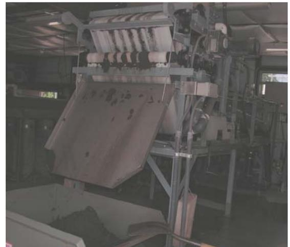
Figure 2: Sludge Cake Belt Press at Patagonia WWTP
